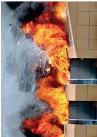
Photo – care of Fire Middle East
