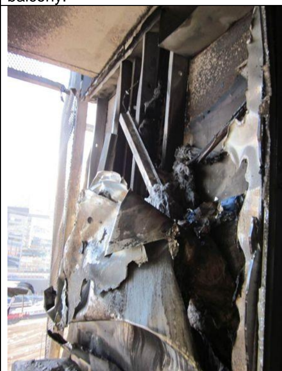
External wall at upper height
