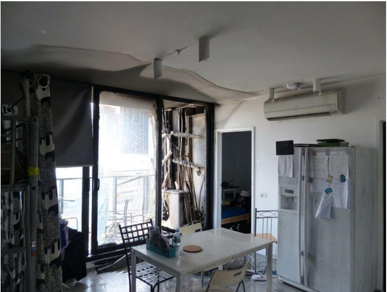
Figure 5 – Picture 4: Inside kitchen looking towards double glass sliding doors leading to balcony area & bedroom 2.
