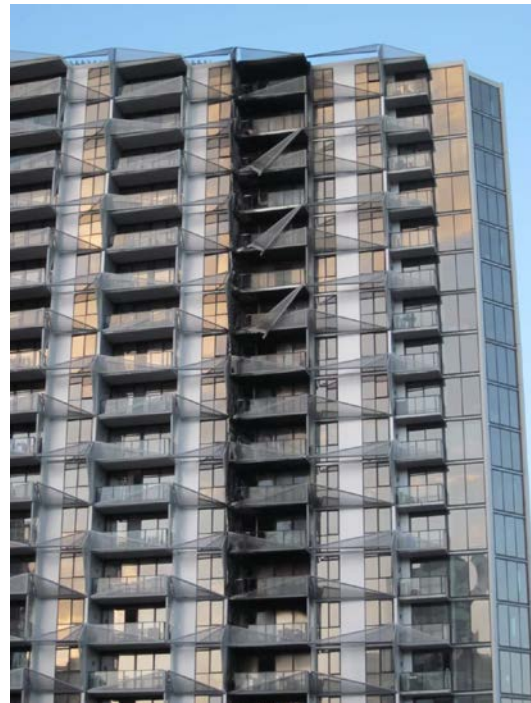
Photo Post Fire
