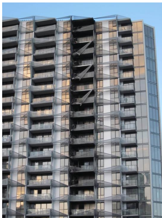
Photo Post Fire
